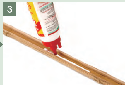
3 Paste glue bonding on the inside of bamboo on all three sides.
